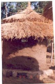
Figure 2: Mud silo (Gotta)
